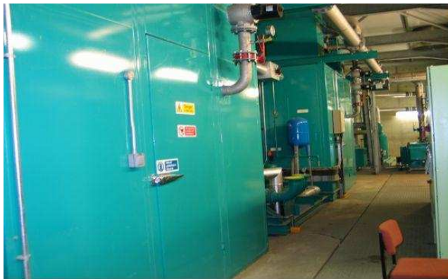
Figure 3: Typical CHP Plant
